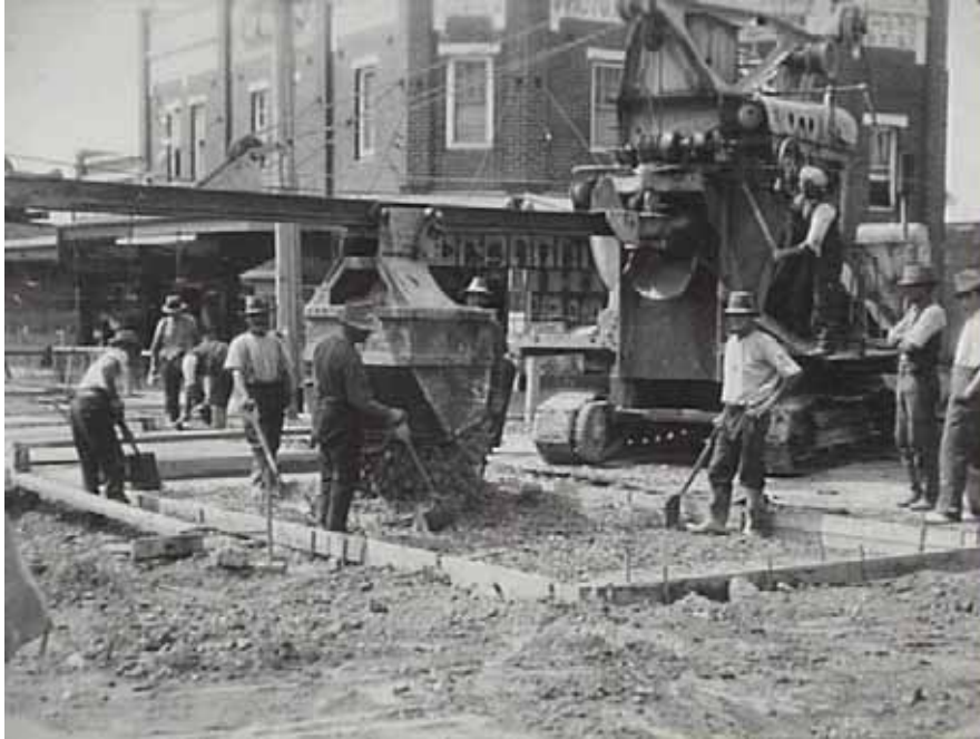
Figure 6-15: Lakemba c.1932, concreting Haldon Street. Source: Bankstown Library Collection via Pictorial Canterbury, item 020201.
