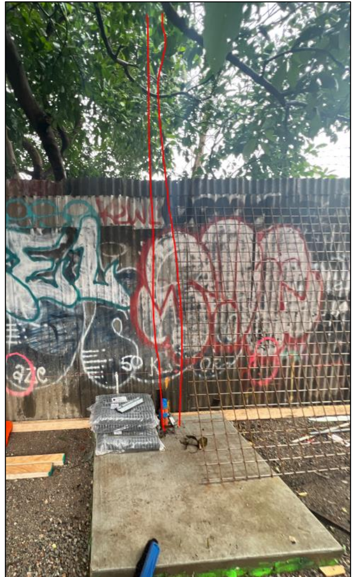
Figure 5: Light post location (Tree 3278)
