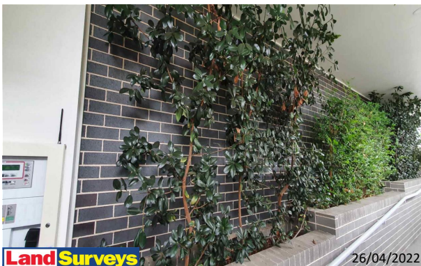
Land Surveys 4 Broughton Street Facades Overview
