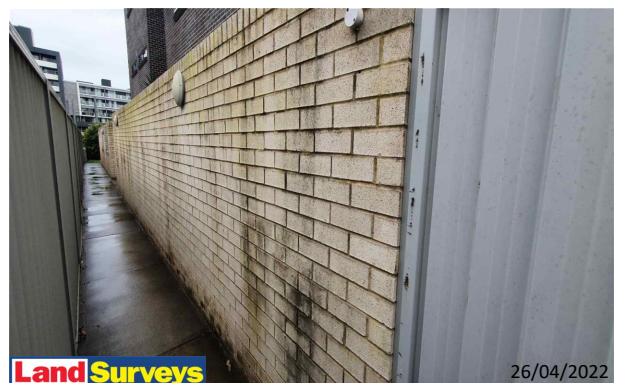
8 Broughton Street Facades Overview
