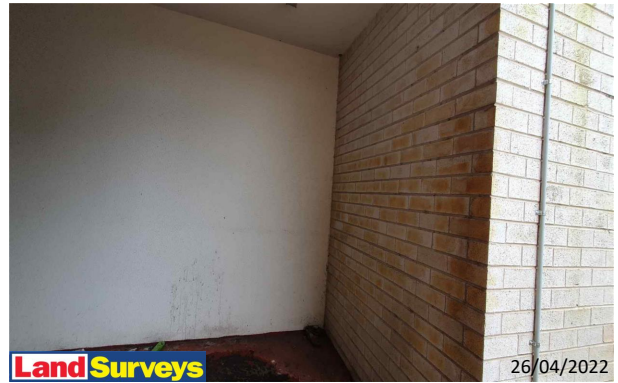
8 Broughton Street Facades Overview
