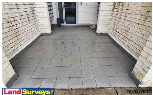
8 Broughton Street Facades Overview
