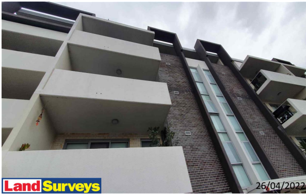
8 Broughton Street Facades Overview
