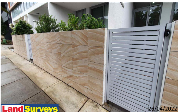
4 Broughton Street Facades North Tile - Cracking - Lineal - 1-5mm - Class 2
