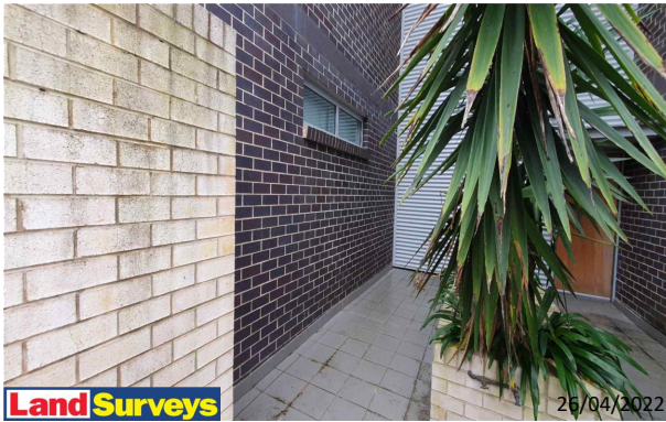
8 Broughton Street Facades Overview
