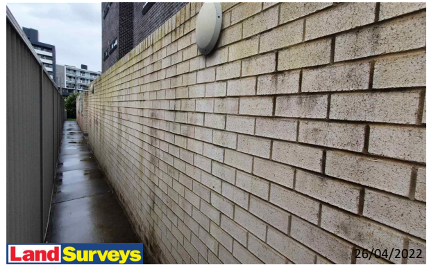
8 Broughton Street Facades Overview
