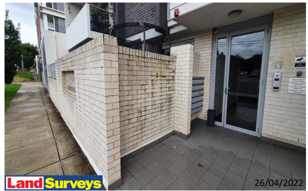
8 Broughton Street Facades Overview
