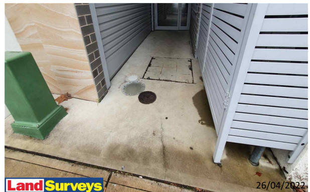
4 Broughton Street Facades Floor Level Slab - Cracking - Lineal - 1-5mm - Class 2
