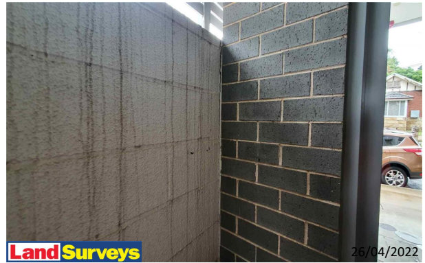
4 Broughton Street Facades North Wall - Cracking - Joint - 1-5mm - Class 2
