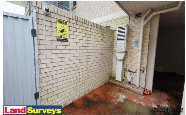
8 Broughton Street Facades Overview
