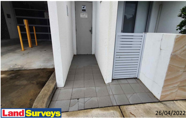
4 Broughton Street Facades Floor Level Tiles - Cracking - Lineal - 1-5mm - Class 2
