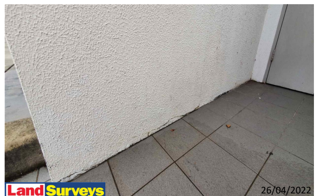
4 Broughton Street Facades East Wall - Cracking - Horizontal - 1-5mm - Class 2
