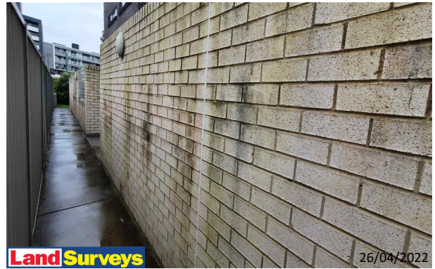
8 Broughton Street Facades Overview
