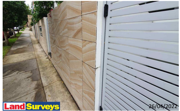
4 Broughton Street Facades West Wall - Cracking - Horizontal - 1-5mm - Class 2
