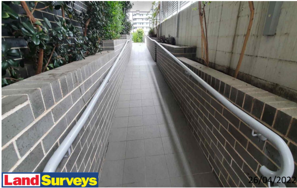
Land Surveys 4 Broughton Street Facades Overview
