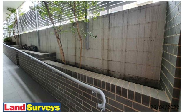
Land Surveys 4 Broughton Street Facades Overview
