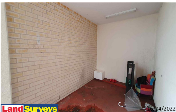
8 Broughton Street Facades Overview
