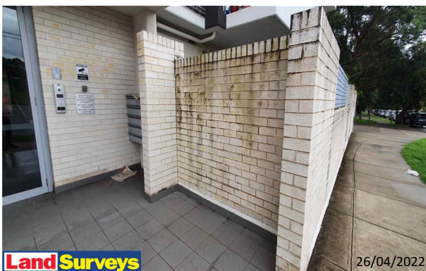
8 Broughton Street Facades Overview
