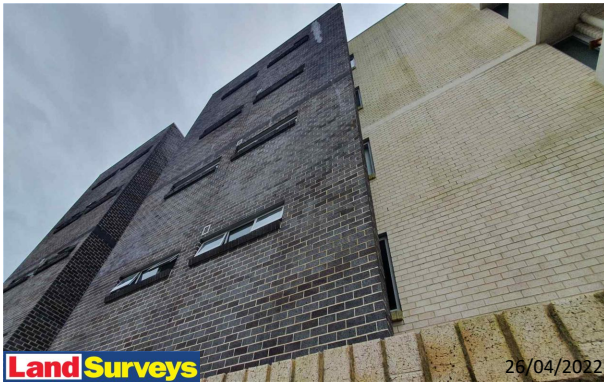
8 Broughton Street Facades Overview
