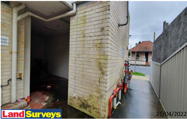
8 Broughton Street Facades Overview
