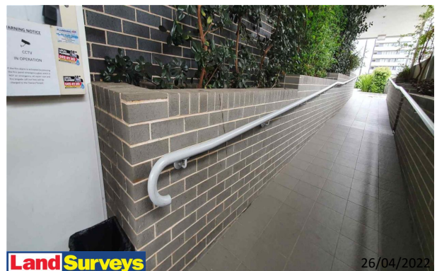
Land Surveys 4 Broughton Street Facades Overview
