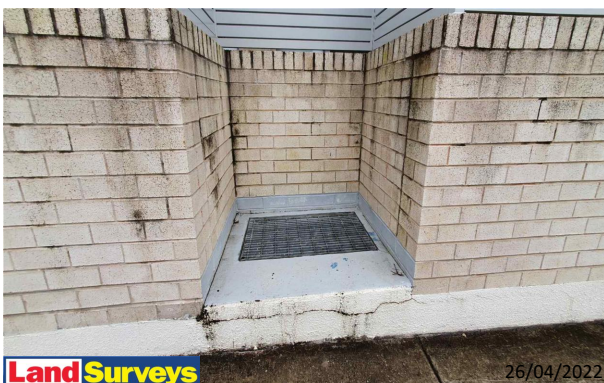
8 Broughton Street Facades Floor Level Step - Cracking - Lineal - 1-5mm - Class 2
