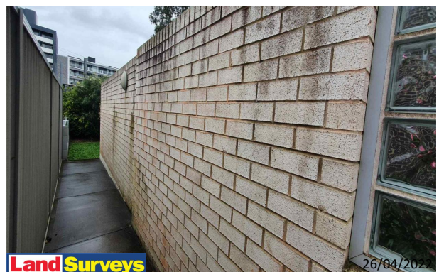
8 Broughton Street Facades Overview
