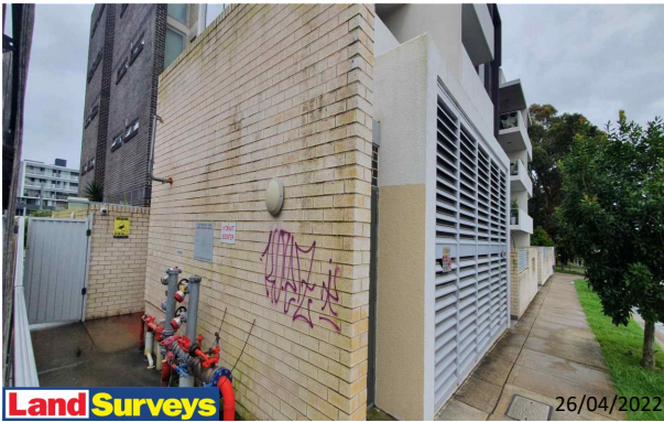
8 Broughton Street Facades Overview
