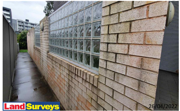
8 Broughton Street Facades Overview
