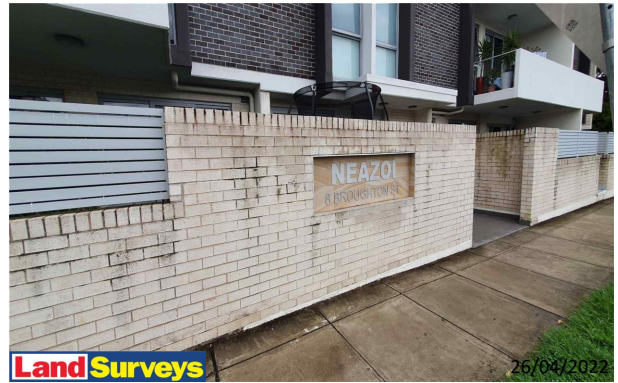
8 Broughton Street Facades Overview
