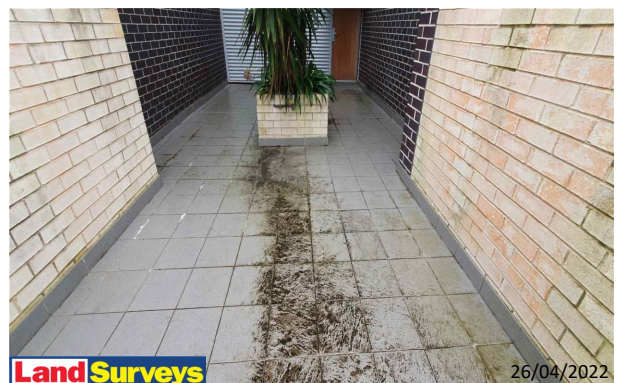
8 Broughton Street Facades Overview
