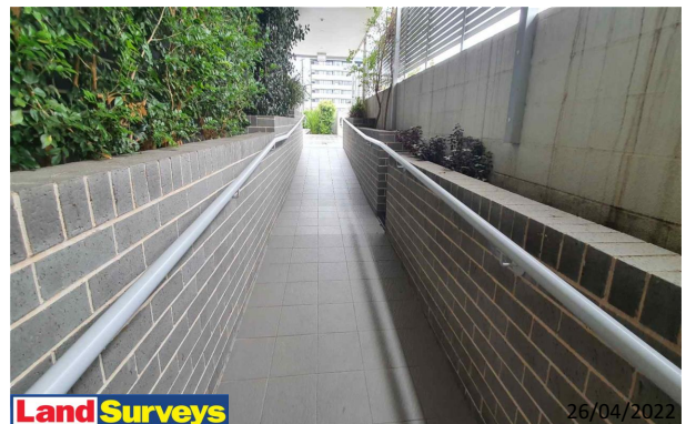
Land Surveys 4 Broughton Street Facades Overview
