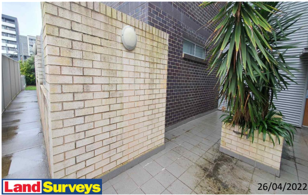
8 Broughton Street Facades Overview
