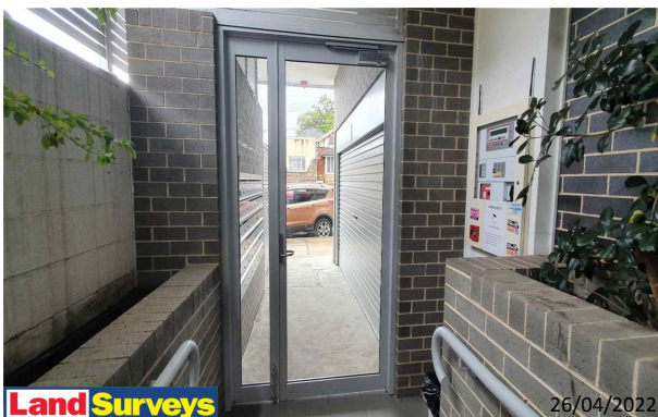
Land Surveys 4 Broughton Street Facades Overview
