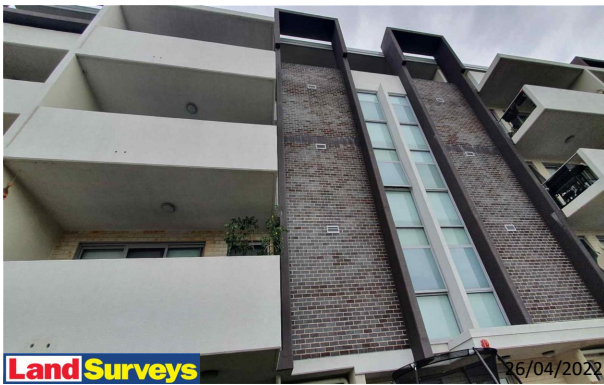
8 Broughton Street Facades Overview
