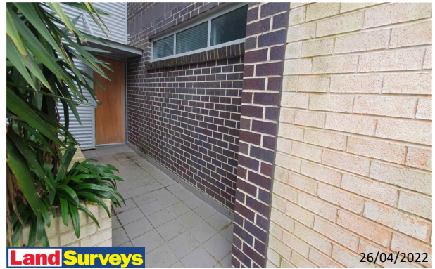
8 Broughton Street Facades Overview
