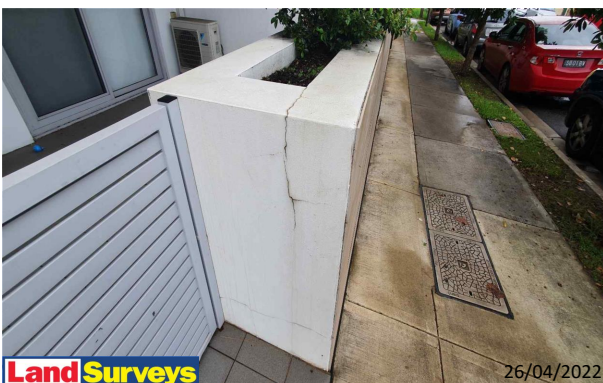
4 Broughton Street Facades East Wall - Cracking - Various - 1-5mm - Class 2
