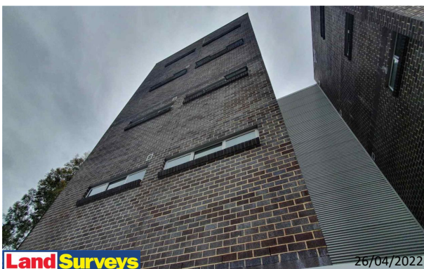
8 Broughton Street Facades Overview
